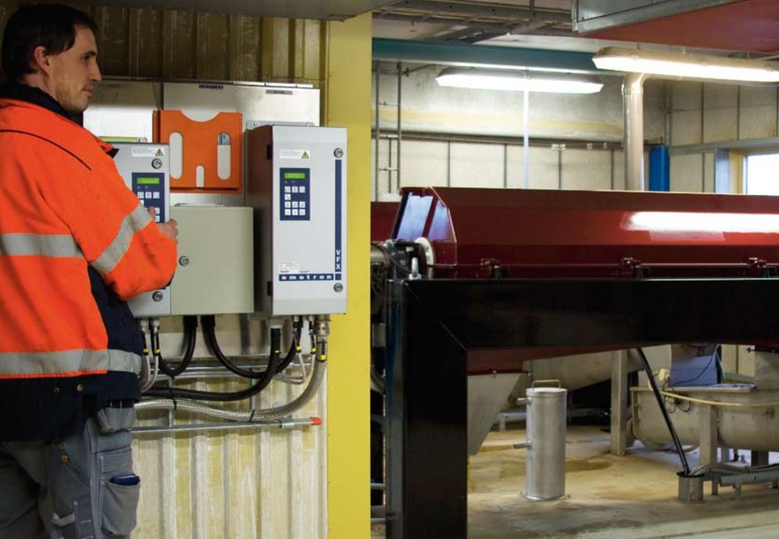
*When Falkenberg treatment plant invested in new equipment for dewatering sludge, they chose decanter centrifuges from Noxon controlled by Emotron VFX variable speed drives. Operational electrician Tomas Bjurklint is happy with the cost-effective solution, with the energy generated by the braking motor being re-used by the drive motor.*
