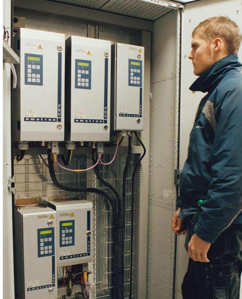
*The plant’s eleven Emotron FDU variable speed drives are installed in an electronics room. Having them all in one place facilitates control and monitoring, according to operating technician Oskar Österling.*
