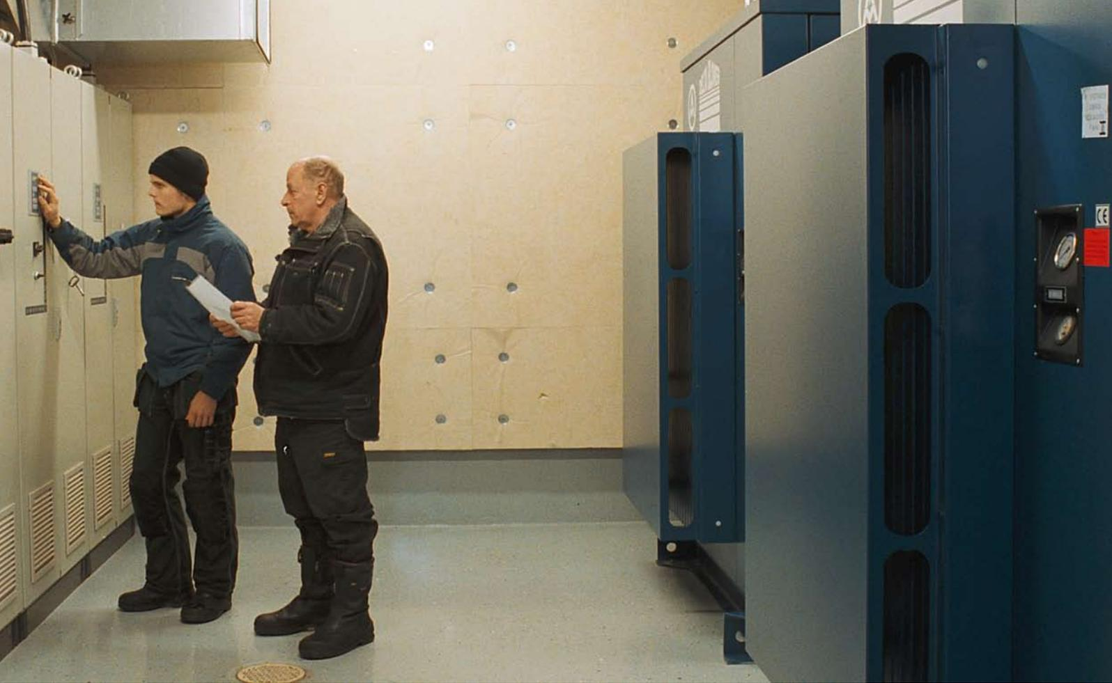
*Emotron FDU variable speed drives control blowers and pumps at Elmo Leather's new wastewater treatment plant. "This is the first time a fully biological purification method has been used in the tanning industry," explains works engineer Jan-Allan Hasselqvist (on the right).*
