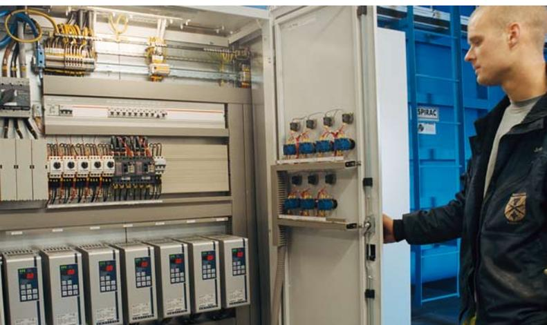
The sludge is dewatered in centrifuges, the screw conveyors for which are controlled by seven Emotron MSF softstarters. The sludge is then used as fertiliser or sent for final disposal.
