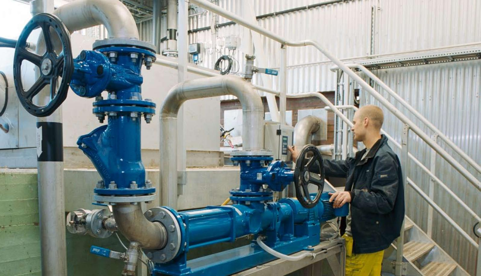
Johan Arvidsson, electrician at the Svenljunga sewage treatment plant, supervising an excentre pump pumping sludge to a thickener. The pump is controlled by an Emotron FDU variable speed drive. An Emotron M20 shaft power monitor ensures nothing is blocking the screw conveyor. "One advantage of Emotron products is that they can withstand harsh environments and be located within the plant, without the need for costly cables or cabinets."
