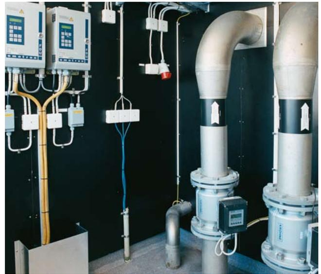
The equipment at the Svenljunga sewage treatment plant used to be controlled manually to a large extent. Today everything is regulated by Emotron products, such as these inlet pumps.
